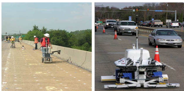
Fig. 1. (Left) Bridge inspection at the Haymarket, VA, USA, testing site. The white dots seen in the image are the bridge deck grid-markings. (Right) RABIT - Robotic Assessment Bridge Inspection Tool: Long Term Bridge Performance (LTBP) program of the Federal Highway Administration (FHWA) [1] has developed a robotic scanning system for imaging bridge decks using nondestructive evaluation techniques (ground-penetrating radar, impact-echo measurements) and high-resolution images. Using this system, we collect image data from bridge decks for developing and testing an automated crack detection algorithm. Path-planning, sensor geometry, and collision detection for the robot scanning are discussed in [2].
