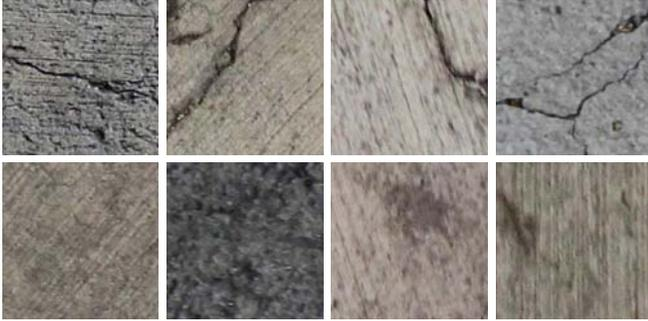
Fig. 4: Images from the “crack” training data (top), and images from the “no-crack” training data (bottom).
