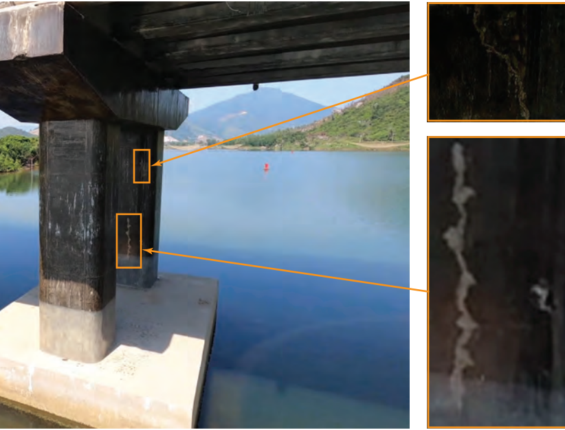
Figure 6. A snapshot from a recorded video taken by the robot. Two zoomed-in areas on the right side show the crack location.
